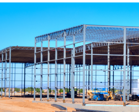
SERVICE AREA CONSTRUCTION
