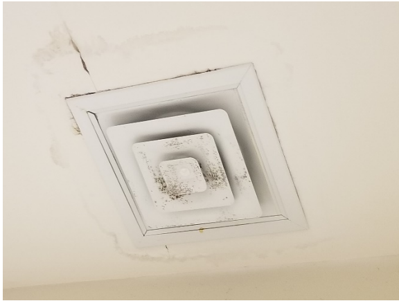
Photo of moisture/condensation stains around supply diffuser due to lack of properly installed insulation.
