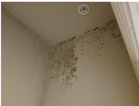
Photo of microbial growth along interior wall of a closet primarily due to vapor pressure diffusion from attic into plenum space above.
