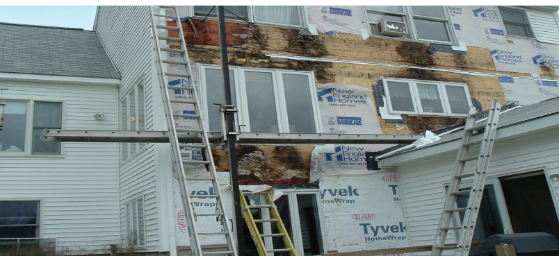
SERVICE AREA ENVIRONMENTAL
