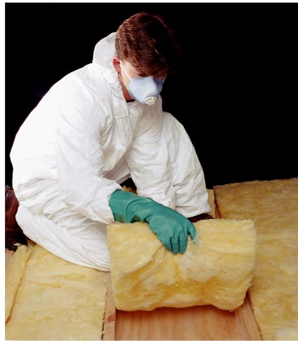
*Fiberglass batt insulation, courtesy CSIRO*
