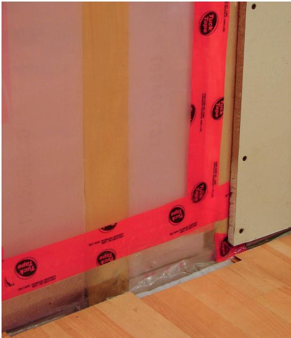
*6 mil Polyethylene plastic sheet as vapor barrier,
