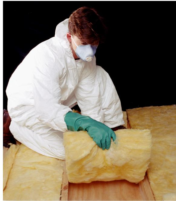
*Fiberglass batt insulation, courtesy CSIRO*
